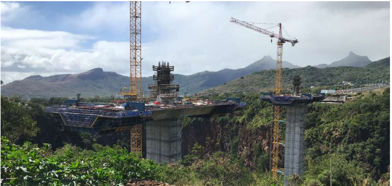
Progress of works on the A1-M1 link
